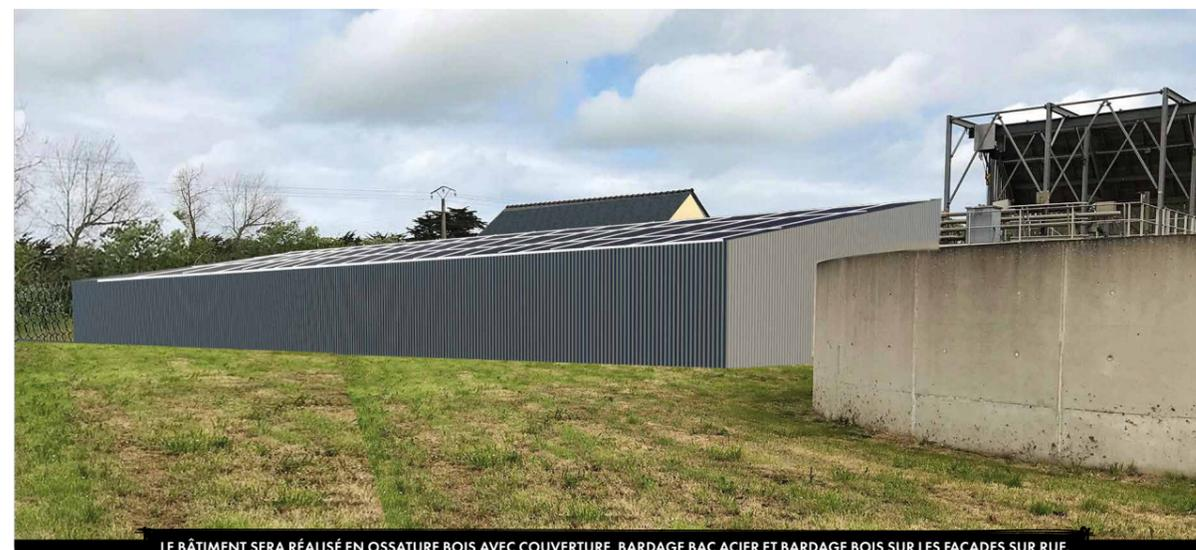
LE BÂTIMENT SERA RÉALISÉ EN OSSATURE BOIS AVEC COUVERTURE, BARDAGE BAC ACIER ET BARDAGE BOIS SUR LES FAÇADES SUR RUE.
